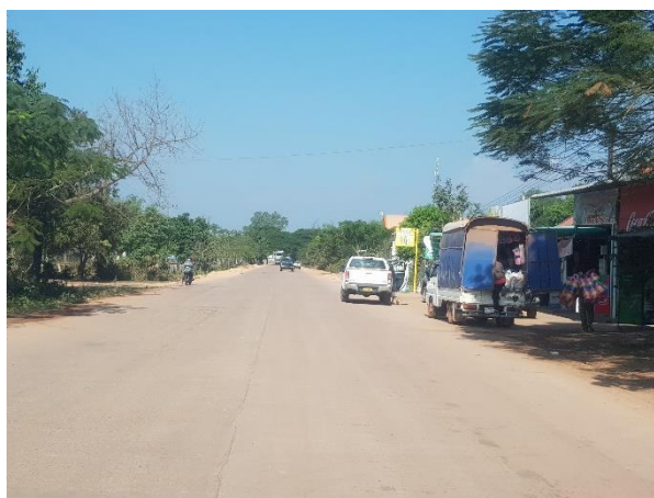
Plate 3-4: Access road to a borrow pit in Ban Donyeng
