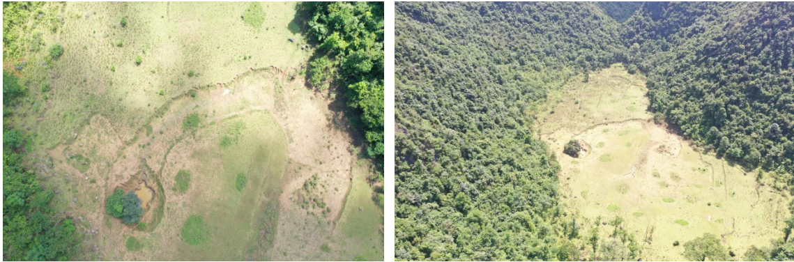
Figure 6.1-4 Current Situation of Bridge Site of Nongwan No. 2 Viaduct
