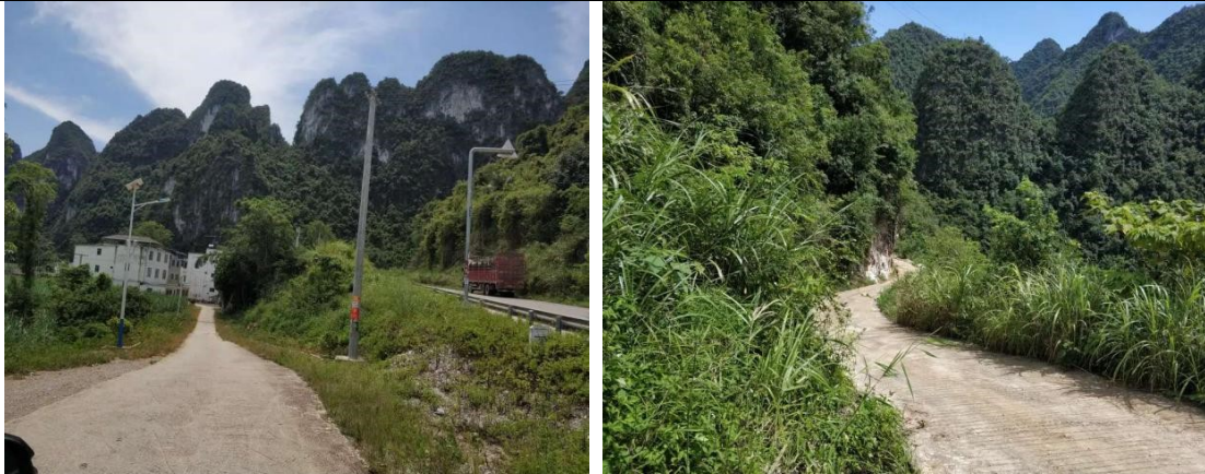
Figure 6.1-17 Village Road to be Widened in K4 Section for Building Access Road
