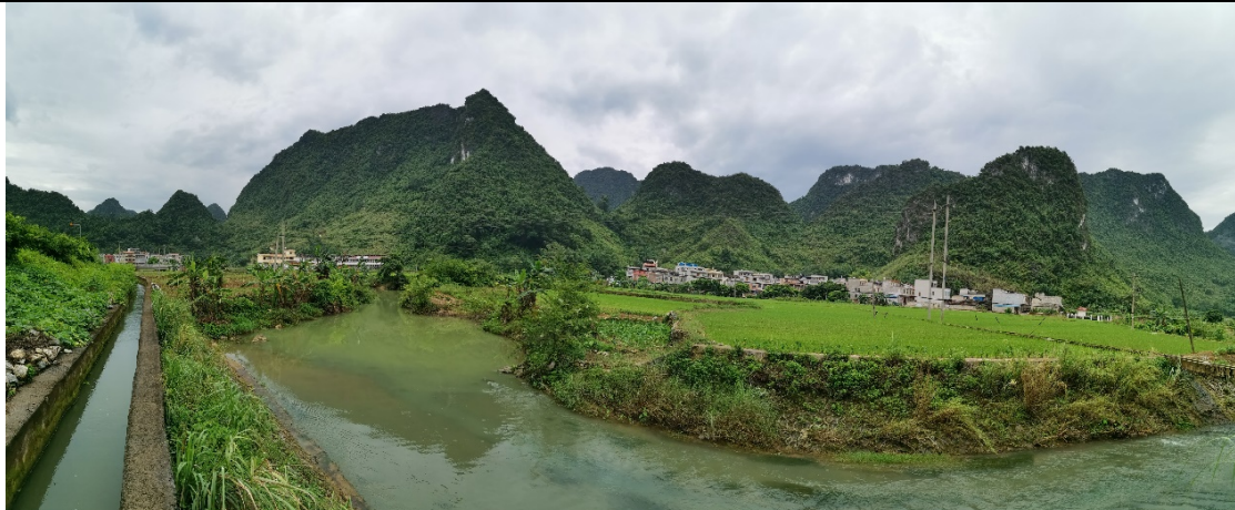
Figure 6.1-5 Current Situation of Bridge Site of Buxuan Viaduct
