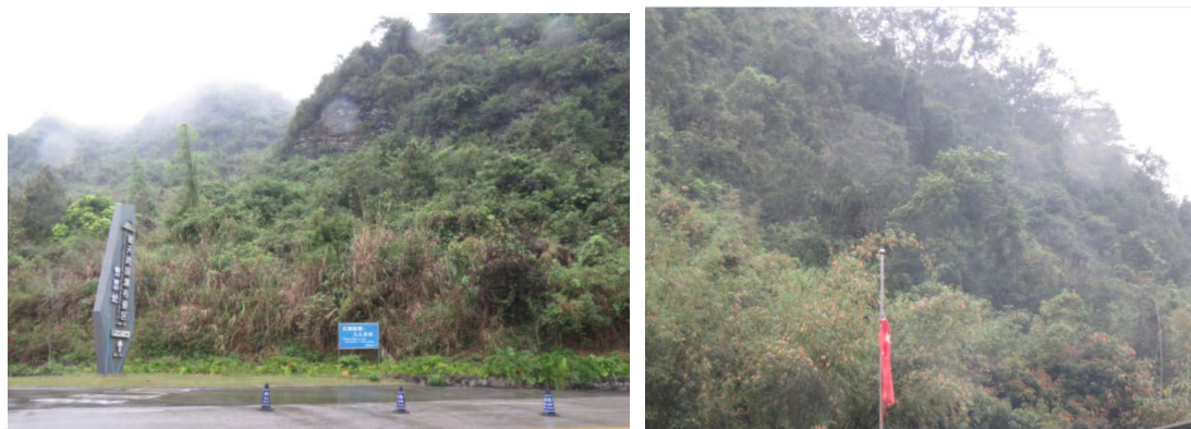
Figure 8.1-5 Project Tunnel Entrance (Left) and Exit (Right)
