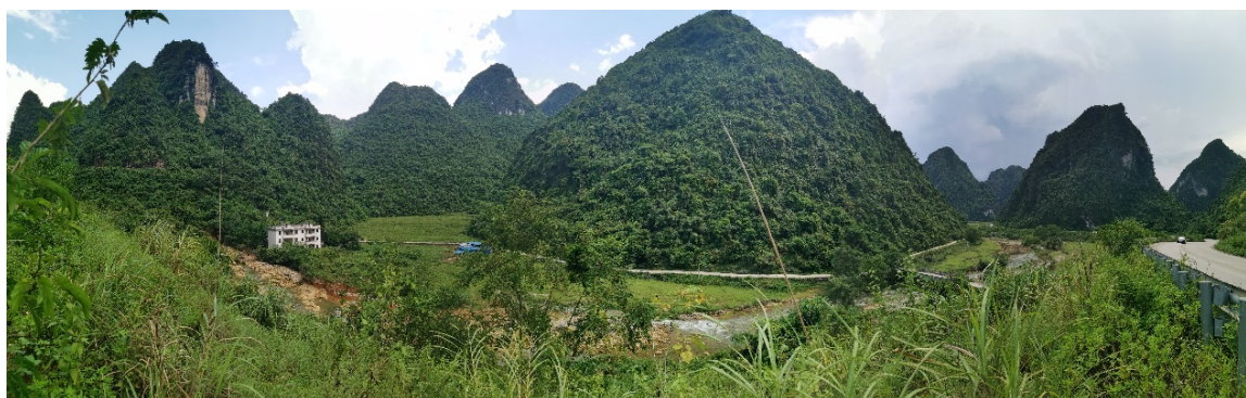
Figure 6.1-7 Current Situation of Bridge Site of Longkalang Super Viaduct
