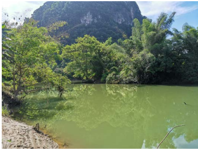
Figure 6.1-8 Current Situation of Bridge Site of Bangtun Heishui River Bridge (7) LZK5+353/ LYK5+337 Shuolong Guichun River Medium Bridge
