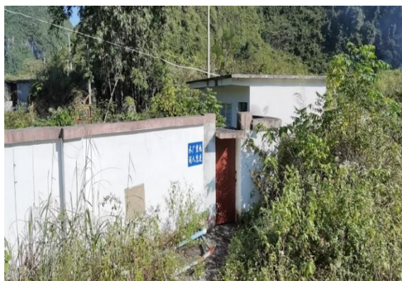
Figure 2-1 Water Source of the Water Plant in Liliang Village, Fuxin Town1
