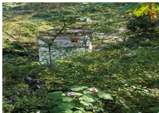
Figure 2-2 Abandoned Building of the Water Plant in Liliang Village, Fuxin Town2
