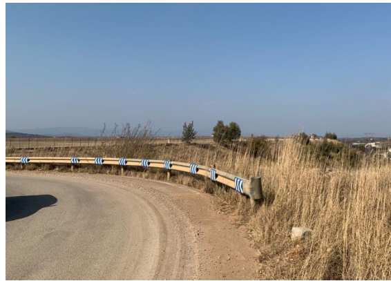
Site of East Runway #2
