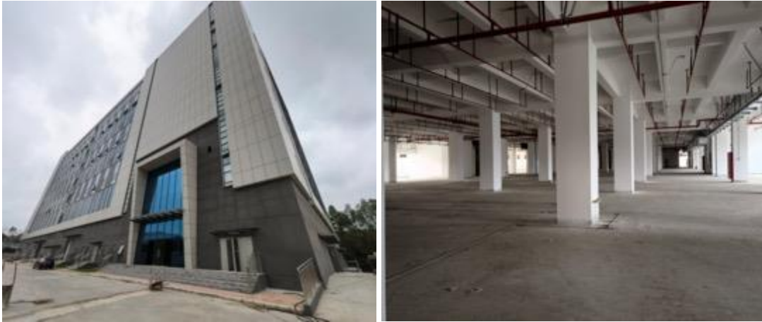
Figure 3-4: Current Site Conditions of the Computational Center
