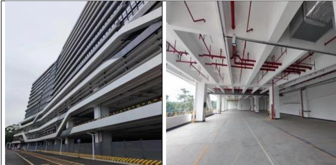
Figure 3-6: Current Site Conditions of the Operations and Management Center and Smart Industry Incubation Platform
