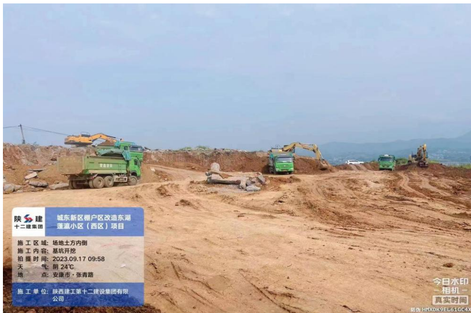
Figure 5-2 Construction Status of Resettlement Community (2023.9)
