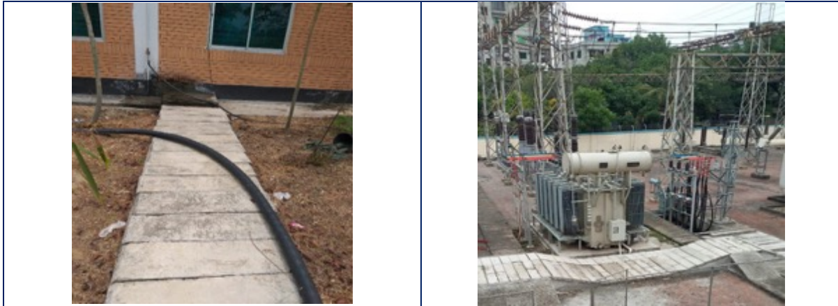
Figure III.14 Underground cable passing through the slab to indoor S/S
