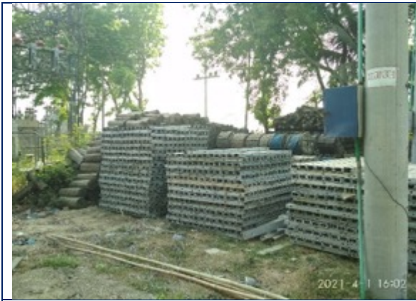
Materials, laying in the substation site at hanail, joypurhat PBS
