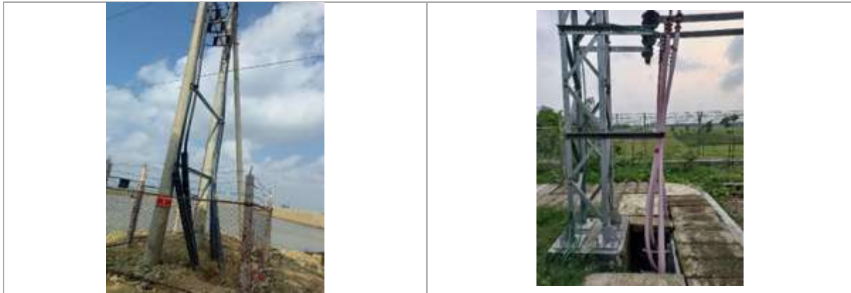
Figure III.17 Underground cable passing through the slab to indoor S/S
