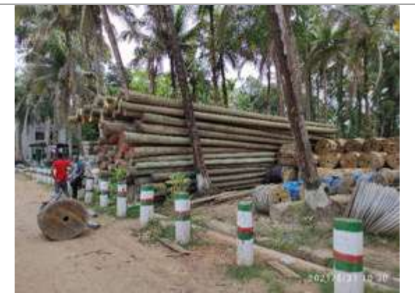
Electric Pole lying in PBS Compound, Laxmipur PBS
