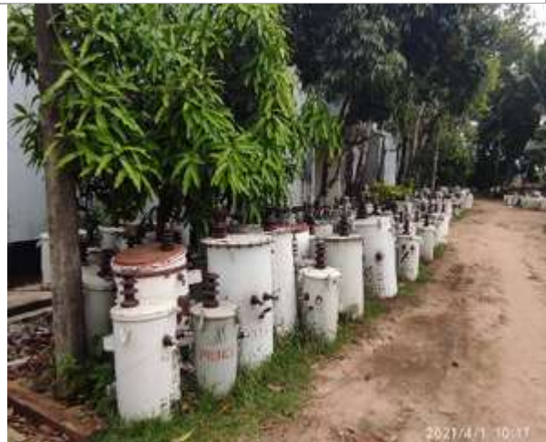
Transformers platform without spill control at Sunamganj PBS
