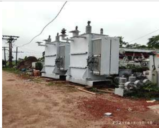
Transformers platform without spill control at Sunamganj PBS
