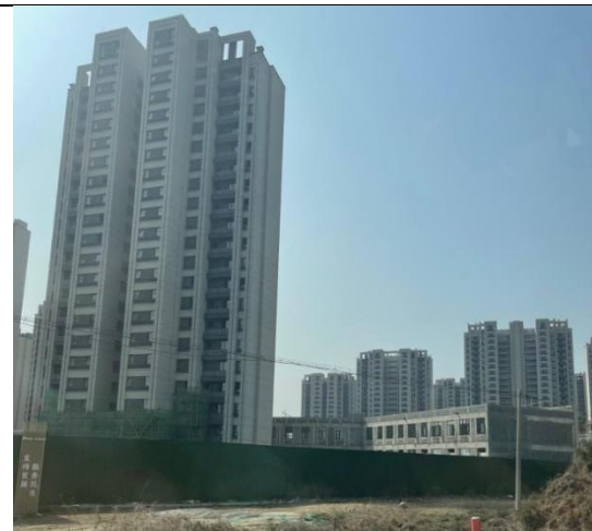
Photo10: Resettlement Area Hechang Jiayuan Construction
