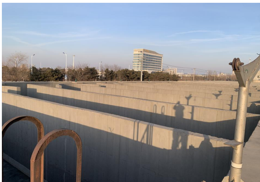
Figure 2-1 Wastewater Treatment Plant
