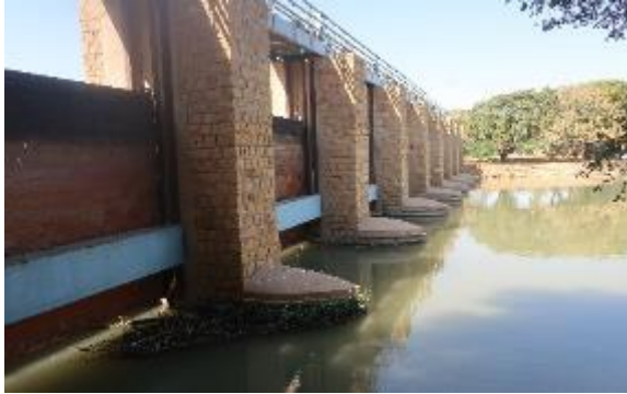
This is the head regulator of Keenjhar Lake at the end of KB Feeder Upper (KBFU) where the water is diverted and controlled to feed Keenjhar Lake, which is built in 1976. The design discharge of the regulator is 8154 cusecs (0.016 MAF per day).
