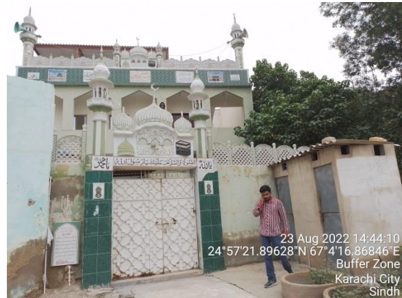
Figure 2-8: View of Mosque Bathroom
