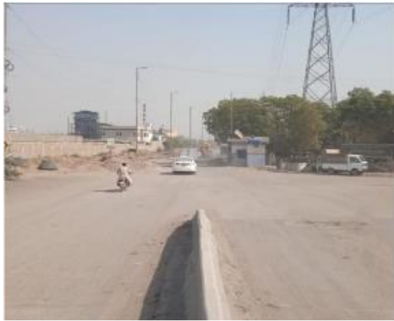
Route-1 from Steel Town Chowk to Qasim Port Rd Bridge (pipeline on the right side of road)
