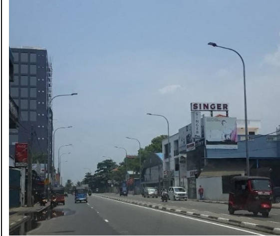
FIGURE 24 View of Improved section of Mattakuliya center Road / Aluth Mawatha - Trench will be excavated at center median on LHS
