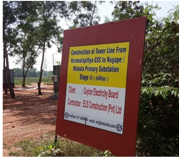
FIGURE 15 Work site for CEB close to the GSS Kerawalapitiya
