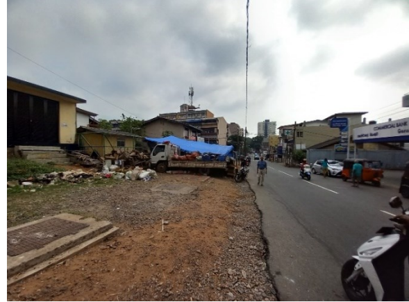
FIGURE 37 Road side to be used for water supply (2024)
