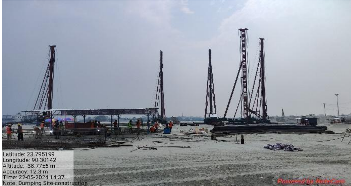
Figure 1-1 Sand piling at Project site
