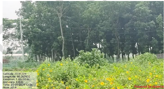
AP-9 Transmission Tower
