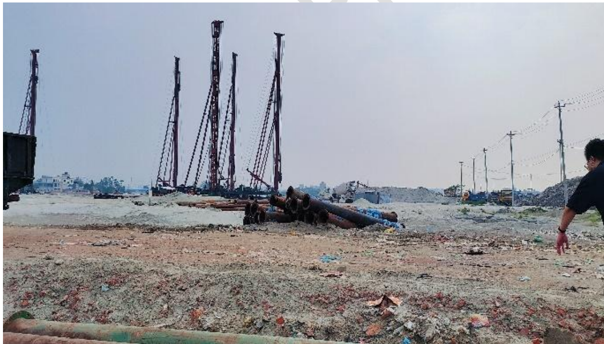
Figure 1-2 Sand piling at Project site
