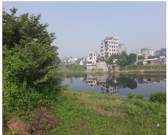
Tower to River Bank Distance (10 m)
