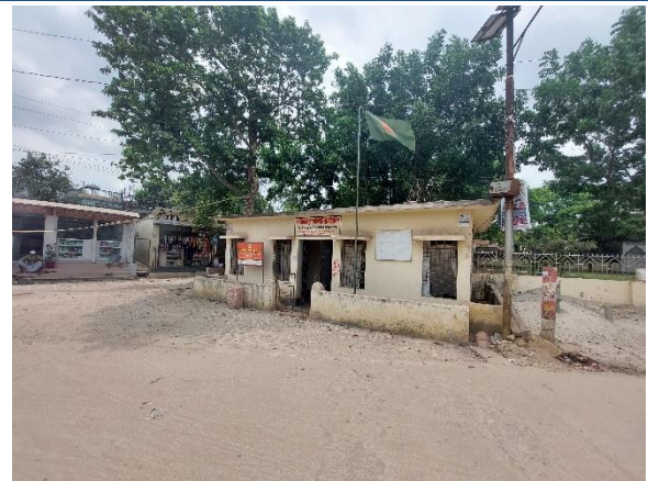
Baliarpur community clinic (approximately 950m North-West directions from the Project Site)
