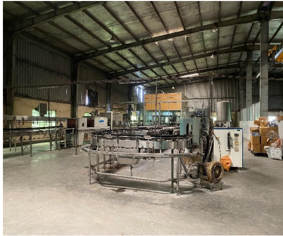
Old Water Plant Machine area
