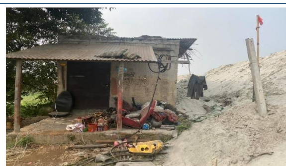
One office room remain after demolishing
