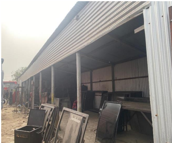
New Storage area
