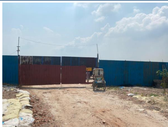
Entrance of New Site with fencing
