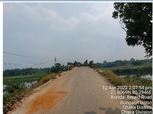
Konda-Beraid Road (approximately 1.4km North-West direction from the Project Site)
