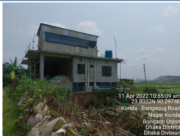
Settlement at the Around 540m north-west side of the project site
