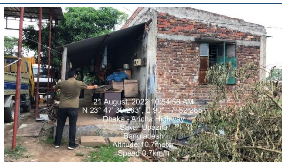
Old Office Before Demolishing
