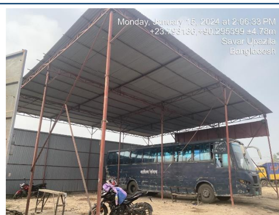
New Shed at new place After Acquisition
