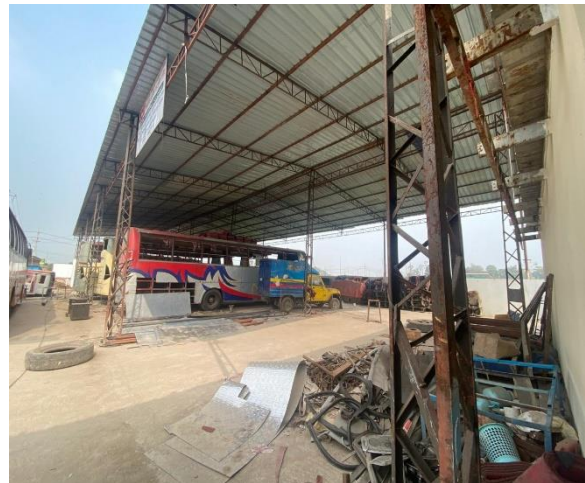
New Repairing Shed
