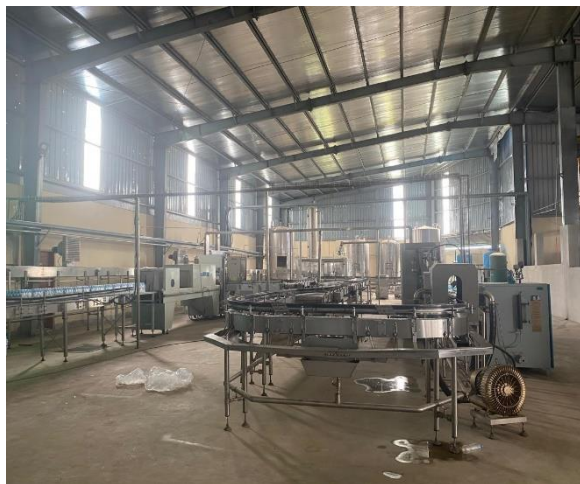
New Water Plant Machine area
