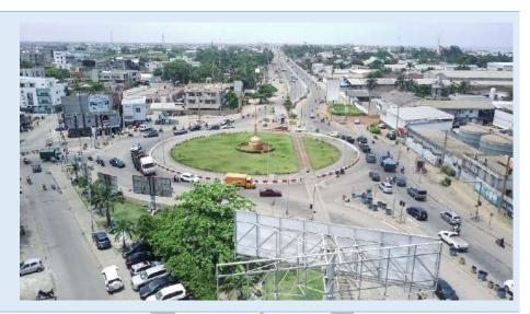
With a roundabout radius of 40m, this intersection is classified as a large roundabout. With a width of 12m for the ring, and an entry and exit lane of 10m; this roundabout is poorly designed and does not meet CEREMA standards. It is decided to:
