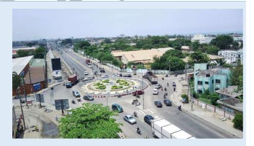
With a roundabout radius of 29m, this intersection is classified as a large roundabout. With a width of 12m for the ring, and an entry and exit lane of 10m; this roundabout is poorly designed and does not meet CEREMA standards. It is decided to:
