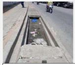
Photo 9: Hole in the Pavement Slab/ risk of removal/ risk of bodily injury to pedestrians
