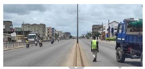
To the left of the double carriageway, there is the presence of the old Cotonou-Sèmè road, currently downgraded as local traffic. Between the local traffic and the main road, there is a railway line whose entire segments of the rails are vandalized and washed away. Between the railway and the main road, there is a metal barrier serving as a separation.
