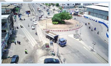
With a roundabout radius of 29m, this intersection is classified as a large roundabout. With a width of 12m for the ring, and an entry and exit lane of 10m; this roundabout is poorly designed and does not meet CEREMA standards. It is decided to:
