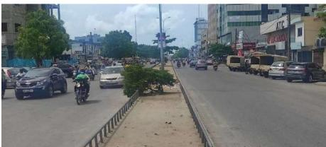
herringbone parking. The sidewalk occupies the rest of the administrative half-right-of-way. Its width varies from 4m to 6m. The gutters are buried on the section from the Carrefour Marché Saint Michel to the Carrefour Marché Missèbo. On the rest of the section, they are visible on the right side. The lighting in the double crosse floor lamp is axial.
