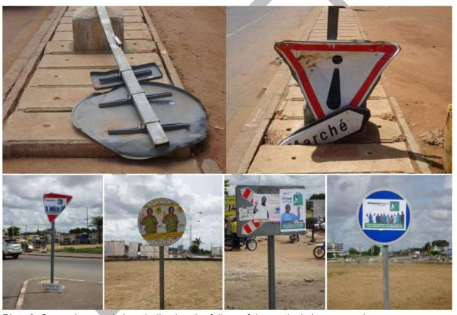
Plate 3: Some damaged signs indicating the failure of the vertical signage on the axes
