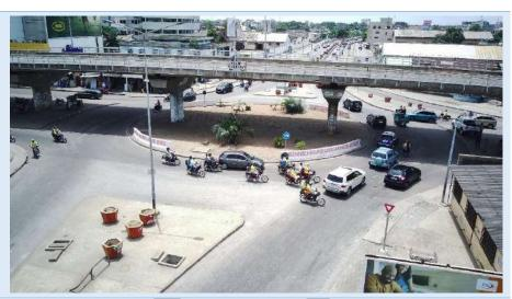
With a roundabout radius of 25m, this intersection is classified as a large roundabout. With a width of 10m for the ring, and an entry and exit lane of 10m; this roundabout perfectly meets CEREMA standards
