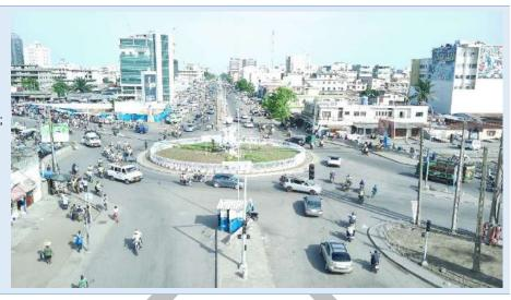
With a roundabout radius of 26.50m, this intersection is classified as a large branches in With a width of 11.50m for the ring, and an entry and exit lane of 10m; that The roundabout is poorly designed and do not meet CEREMA standards. It is decided to:
