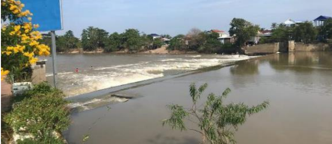
Figure I-3: Kbal Hong Weir (constructed 2018 replacing the old gated regulator)
