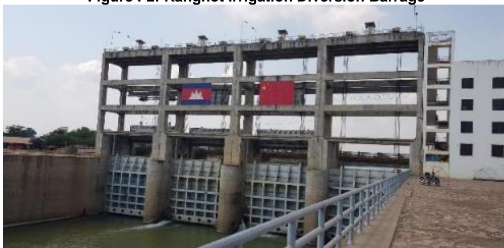
Figure I-2: Kanghot Irrigation Diversion Barrage
