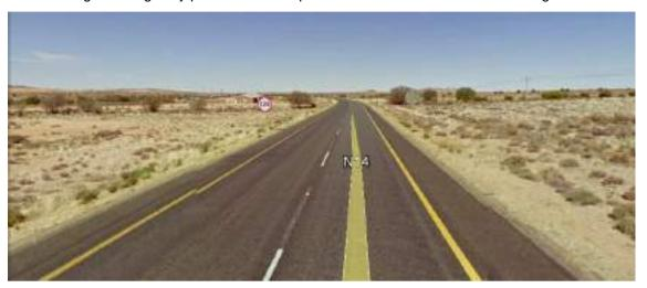
The road is approximately 8 m wide and is located within a 45 m wide road reserve. The speed limit of the road is 120 km/h.
