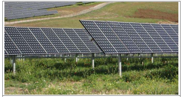
Figure 1: Fixed tilt PV array
