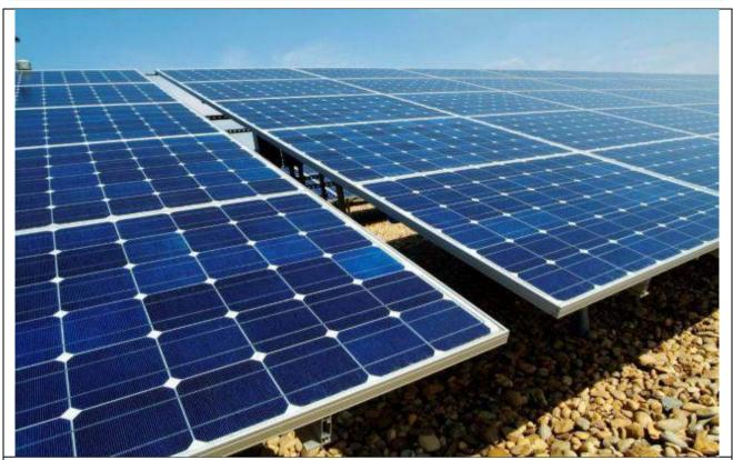
Figure 3-1: Fixed tilt PV array (sourced http://explow.com/solar\_panel)
