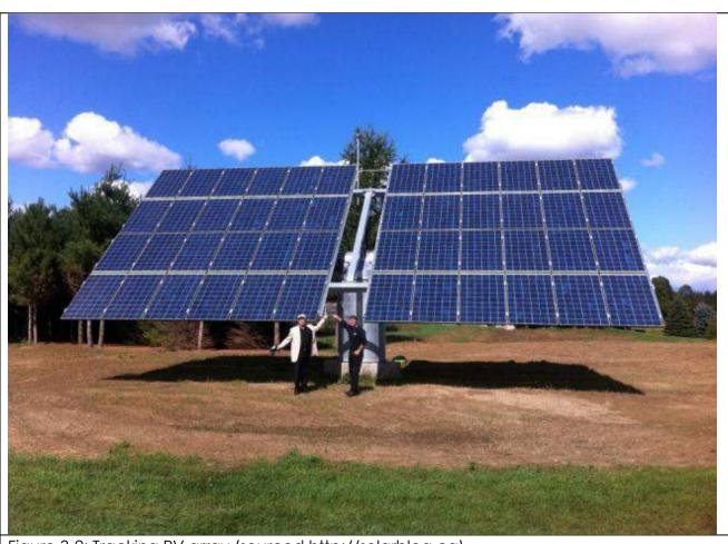
Figure 3-2: Tracking PV array (sourced http://solarblog.ca)
