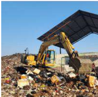
Existing Landfill Condition
