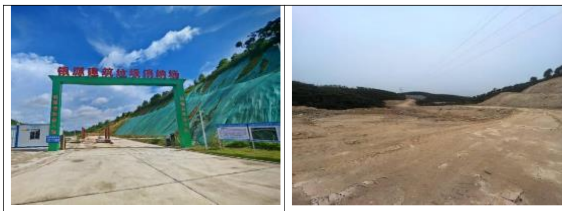
Figure 2: Current Situation of Yinyuan Construction Waste Disposal Site
