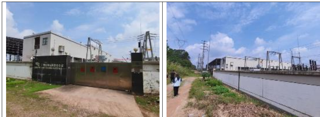
Figure 3: On site Investigation Photos
